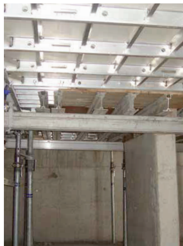
Time-saving Hanging Bracket for column drops
